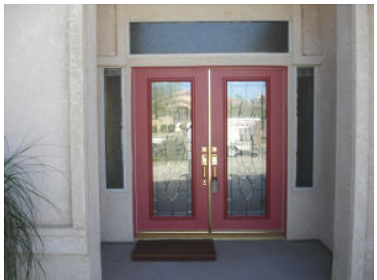
4-New Upgraded Lead Glass Doors Installed
