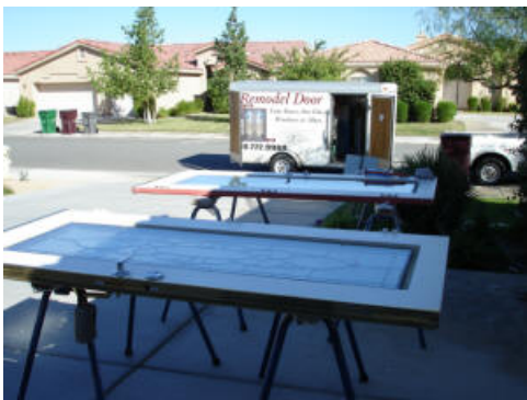
3-Lead Glass Panel Installed
