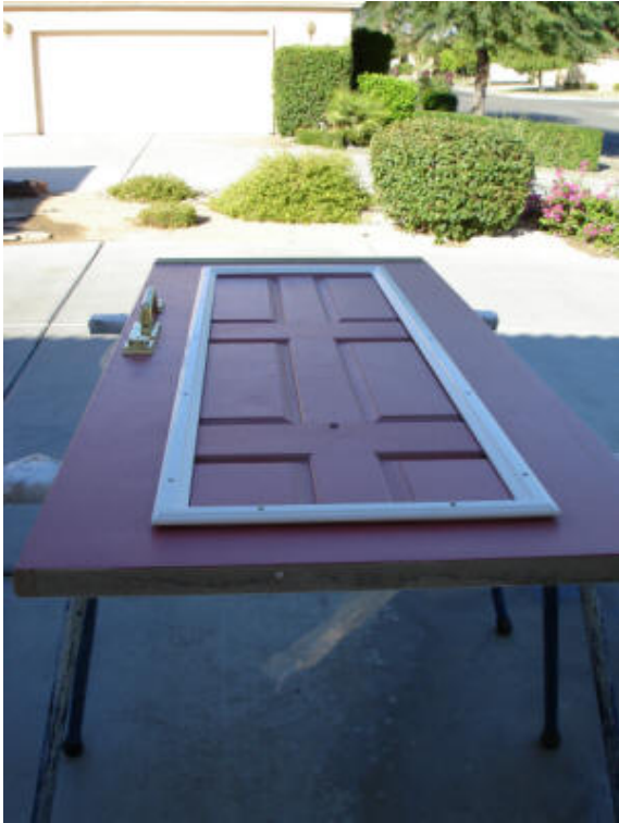
1-Preparing Door For Lead Glass Panel
